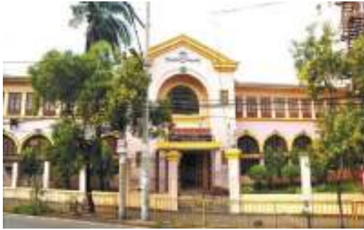
Hugh Wilson Hall Main Building
